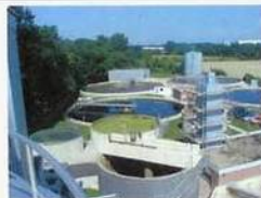
Aeration Tanks, Final Thickener
