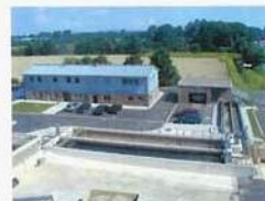
Operational Building – Mechanical Part
