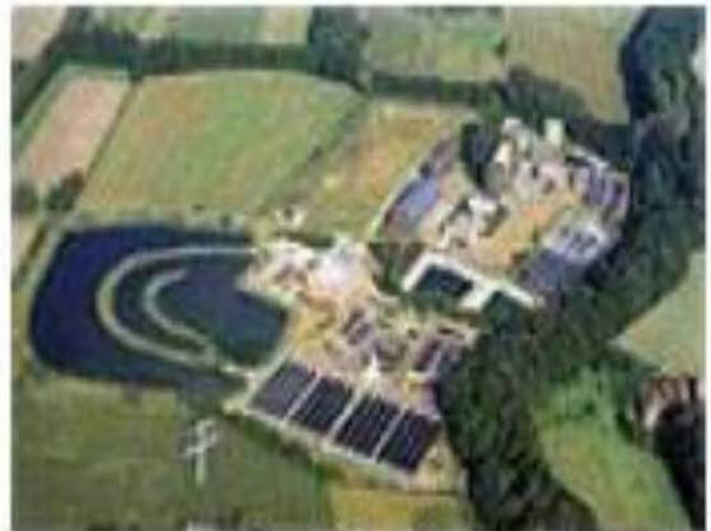
Aerial view Wastewater treatment plant "Obere Lutter"
